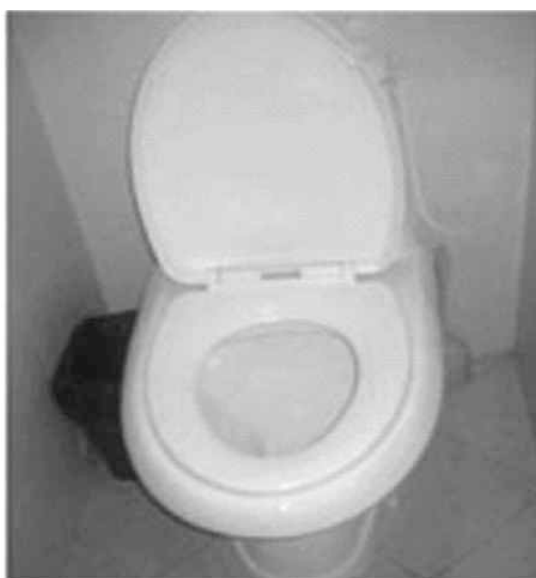
Figure 2.10 Cistern flush toilet cistern or tank is behind the raised lid.
